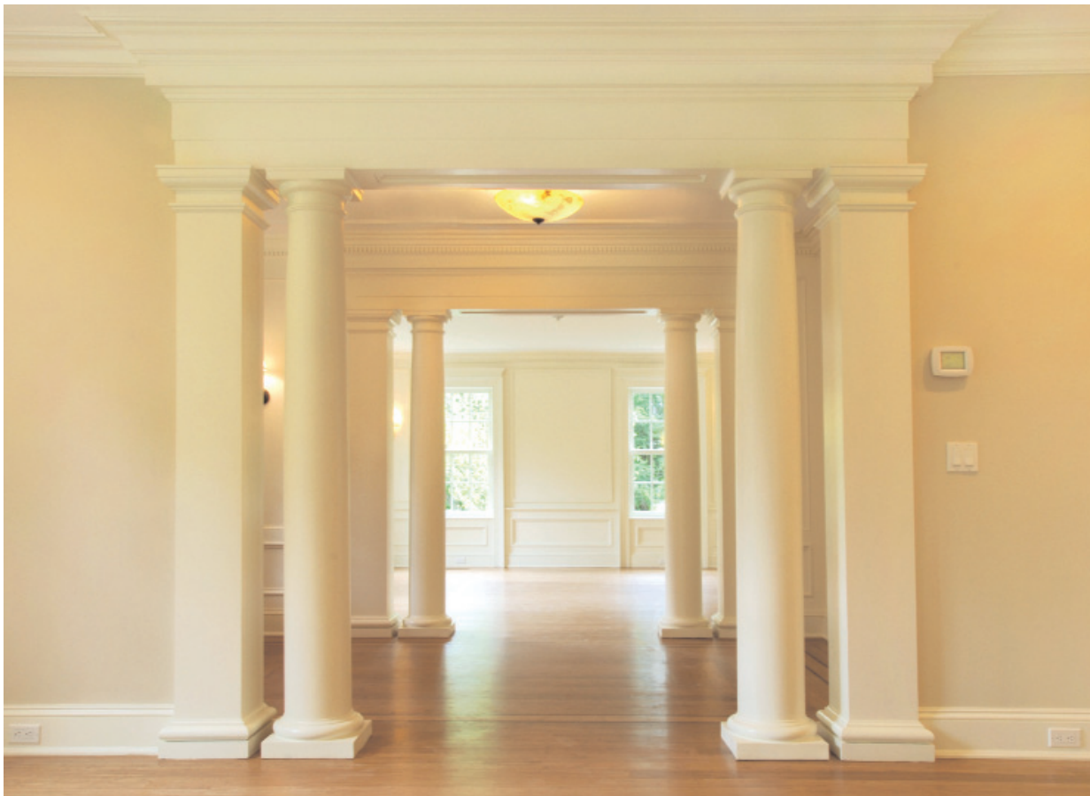
The living room's Classically detailed columns and entablature are seen alongside a programmable digital thermostat that controls the home's geothermal heat pumps.
